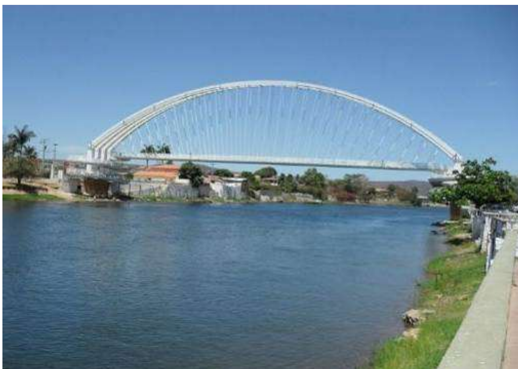
Figure 3.9.9: Footbridge on the Corrente River (stretch 10). (Panoramio, 2013)
