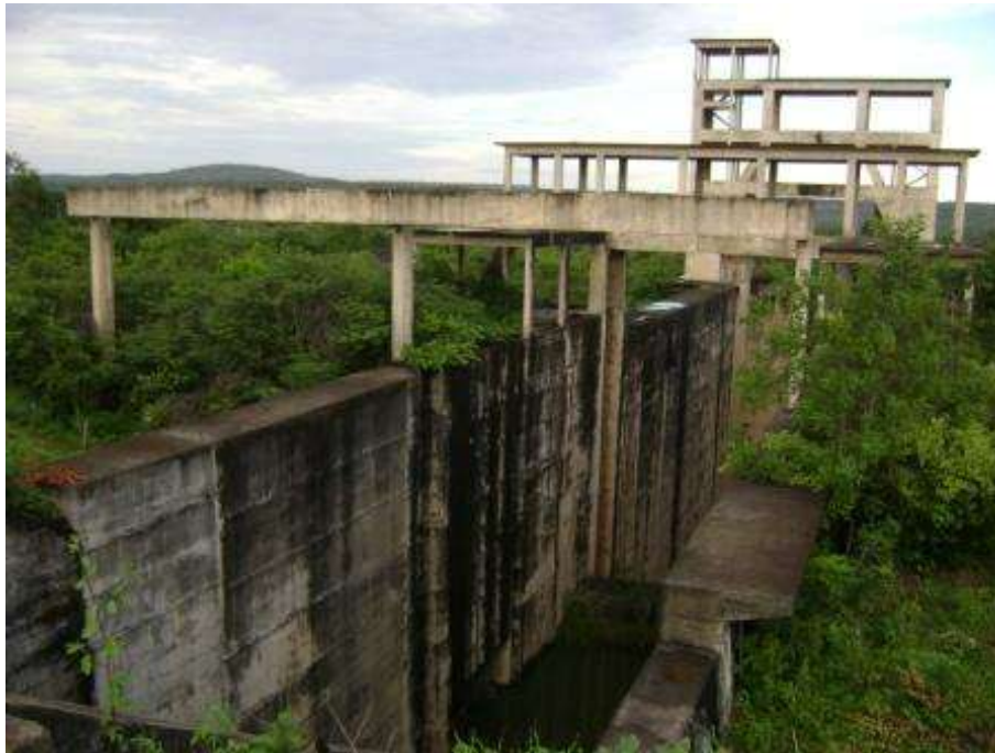
Figure 3.8.2: Unfinished lock at Boa Esperança's hydroelectric plant (Portal Gterra, 2013)
