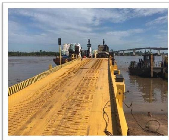
**FIGURA 06 – Rampa *Roll-On Roll-Off***
